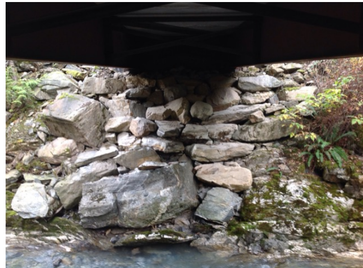
Right Bank Abutment when facing downstream
