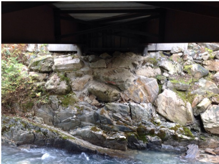
Left Bank Abutment when facing downstream
