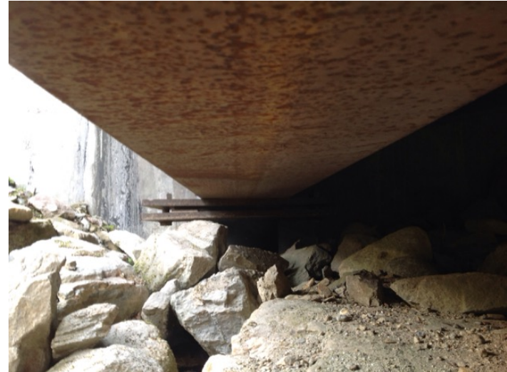
right downstream bearing slightly off center
